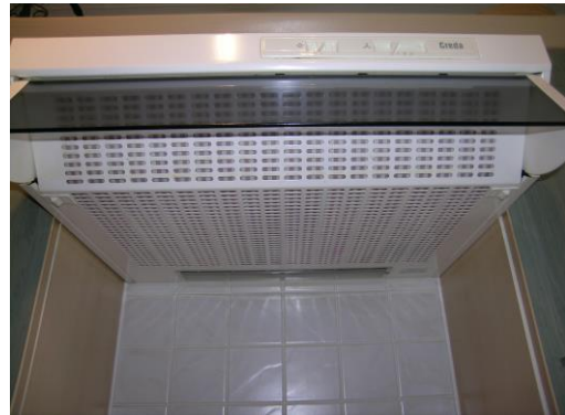
The above is an example of extractor fan – which must be taken apart – and the filter replaced with a new one (bought from any local Hardware shop) – and the white grill cleaned.
